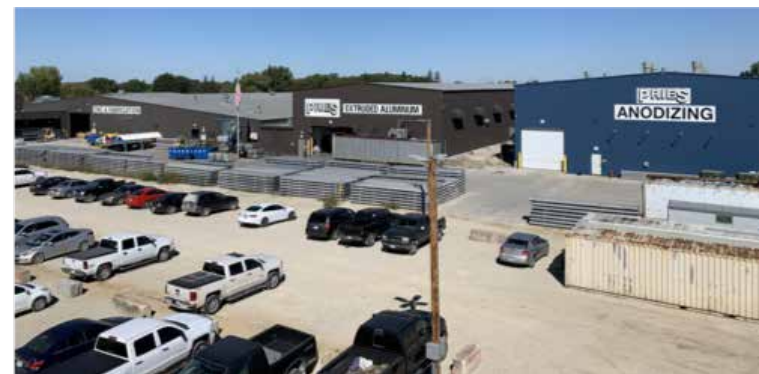
Existing Buildings of Pries Enterprises.
